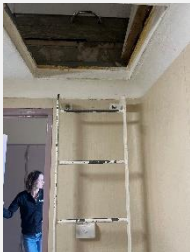
Ladder to roof space
