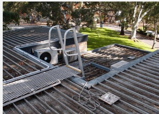
Access to split second level
