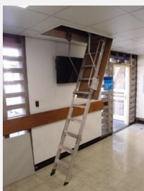
Roof hatch corridor
