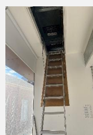
Roof hatch 314a
