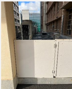
Plant access door
