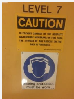
Plant access door
