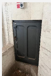
Roof space access
