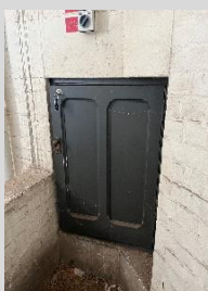
Roof space access
