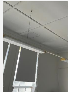
Manhole (RM 108B)
