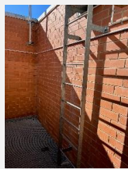
Ladder to upper roof
