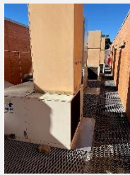
Plant- lower roof
