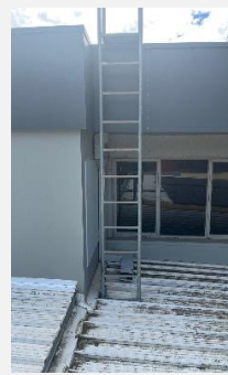
Ladder to upper roof
