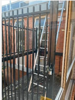
Roof access ladder
