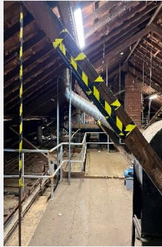
Central roof space
