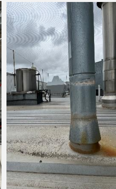
Plant room roof
