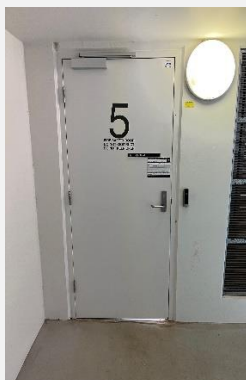
Eastern roof entrance
