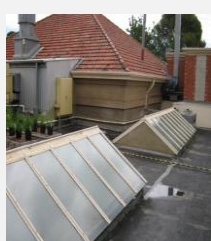
A frame skylights
