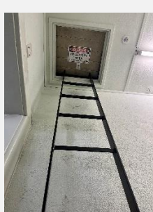
Entry to roof space
