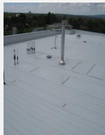
Plant room roof
