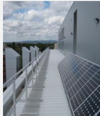
Roof 1 looking east
