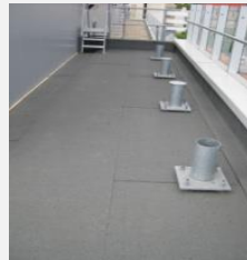
Roof 1 membrane area
