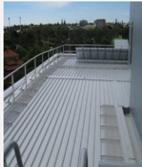
Roof 1 looking north
