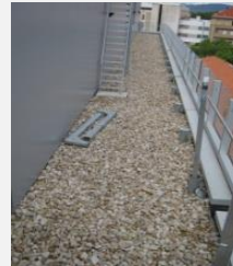
Roof 1 rock area
