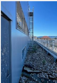
Plant room roof ladder
