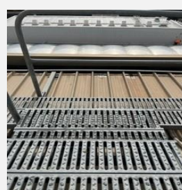
Platform and railing outside hatch
