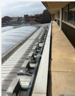
Walkway outside level 7
