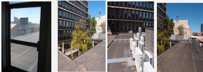
Access door Courtyard Eastern plant Western plant
