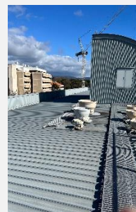
Upper level roof
