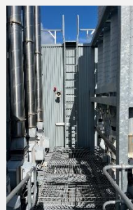
Ladder to upper level
