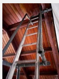
Ladder on platform
