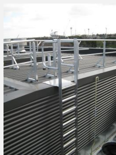
Stairs to lower level of roof
