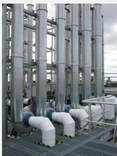
Plant; Western roof
