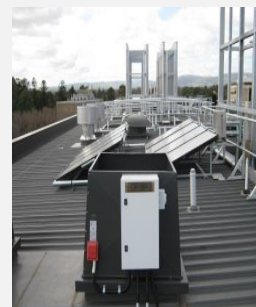
Plant; Western roof
