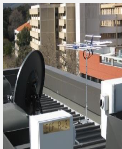
Plant on Eastern roof
