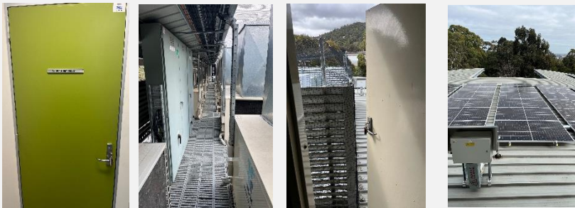
Entrance door Roof platform East side West side
