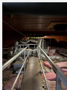
Northern roof space
