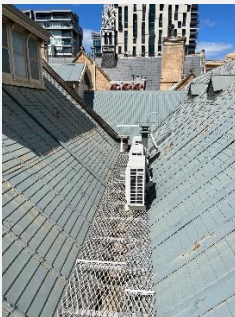
Northern roof walkway
