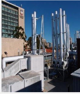
Eastern fume stacks
