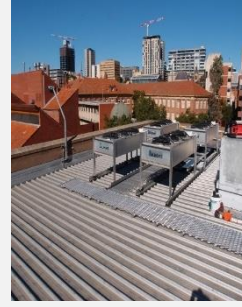
Unprotected edge Eastern side
