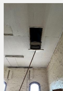
Level 3 - roof hatch
