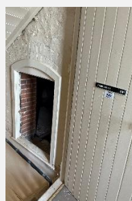
North hatch – level 2
