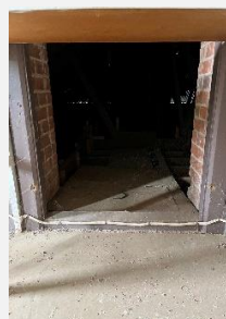
South hatch - level 2
