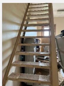
Stairs to level 3
