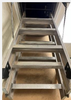
Roof hatch room 112
