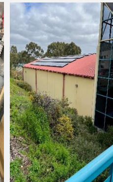
South west roof
