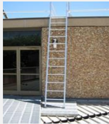
Fixed ladder to Barr Smith South roof
