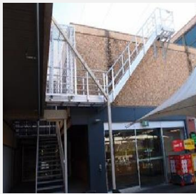
Access from courtyard
