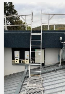
Access to upper roof
