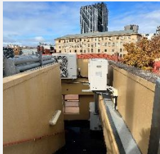
Plant in outdoor stairway
