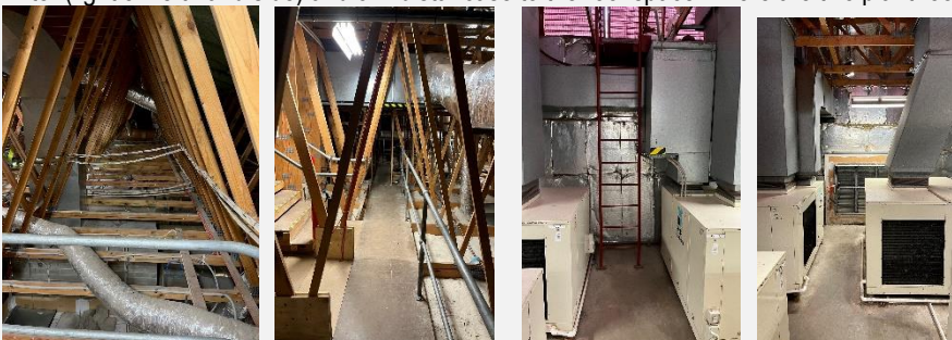
Roof space Walkways Plant in roof space Roof space two
