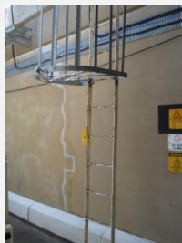
Access to upper roof and warning signs
