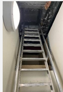
Access ladder & hatch
